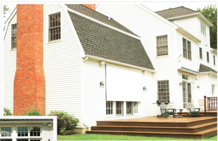
Exterior Solar Shade partially lowered
